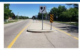
A raised median island is an elevated median constructed on the centreline of a two-way roadway to reduce the overall width of the adjacent travel lanes.
