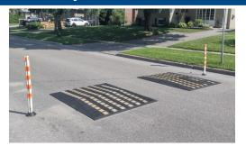
Speed Cushions are two or more raised areas placed laterally across a roadway with gaps between the raised areas to facilitate emergency vehicles. Their application is primarily on local and collector streets at mid-block locations.
