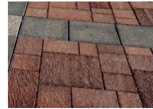
Decorative Paving, Preferred: Unit paver, random pattern, minimal texture, blended red/brown colour.
