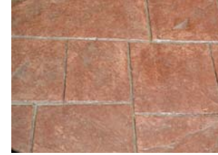
Alternative Decorative Paving: Stamped concrete, random pattern, blended red/brown colour.
