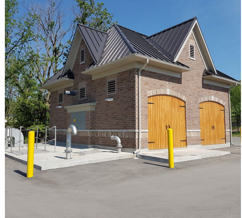
Example of enhanced architectural elements at McClung Sewage Pumping Station
